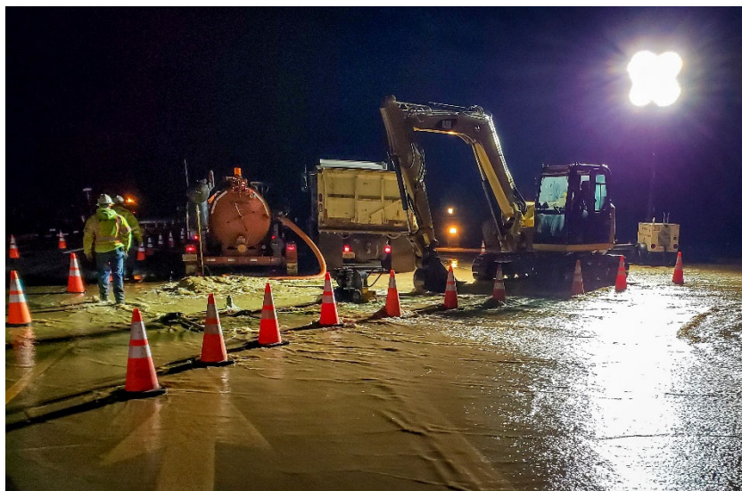
Above: Treated Water Maintenance crews prepare to isolate and make repairs to a 12-inch PCS main break in Rocklin Road.
