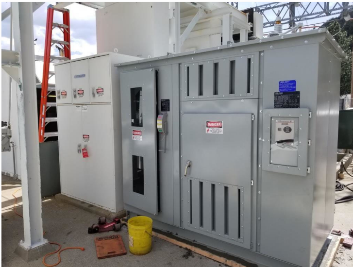
The French Meadows Power House generator excitation transformer and disconnect switch, shown here.
