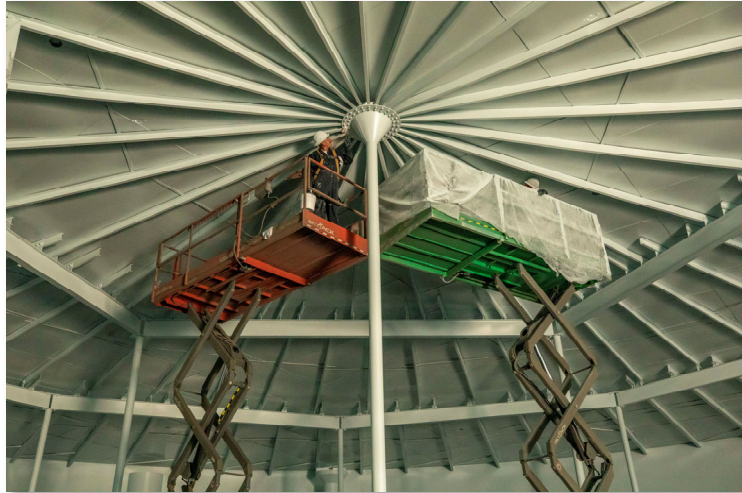
The interior of the Sunset Tank was recoated to prevent rust and corrosion.
