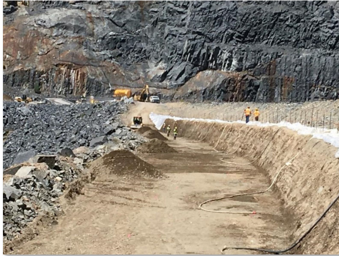
In order to raise the clay core, crews had to excavate about 30 feet off the top of the dam to reach the existing core.
