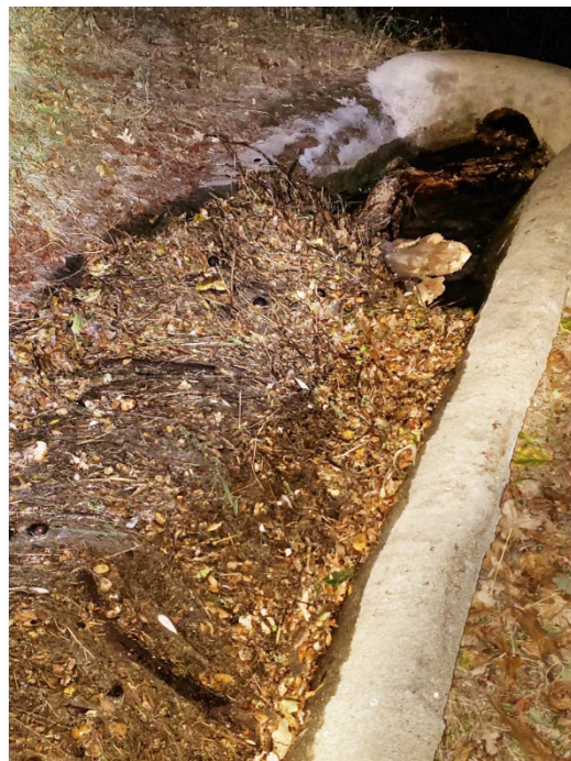
This section of the Shirland Canal was clogged with debris after water flows resumed, following a strong winds during PG&E's PSPS event in late October.
