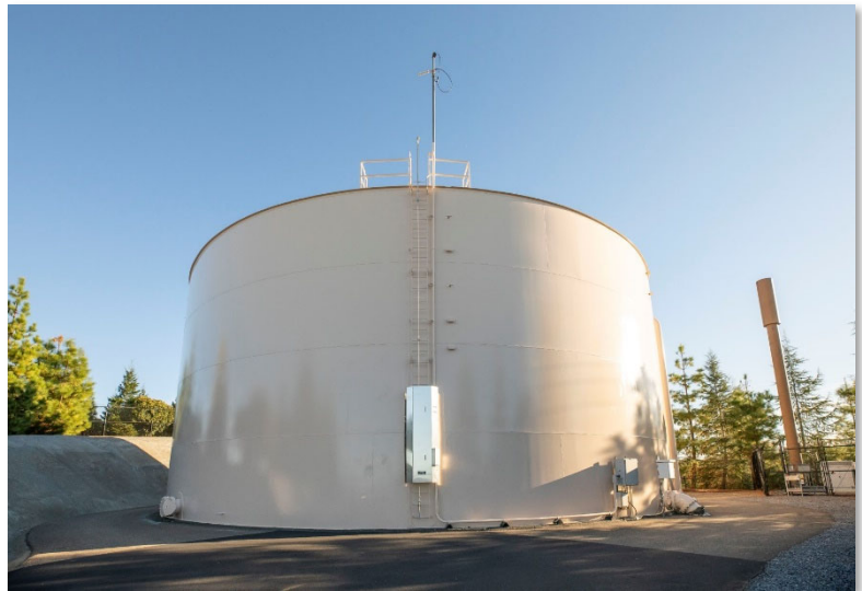
The Rocklin Road Tank was recoated to extend its useful life.
