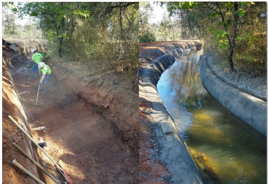
Left: Crews prepare a section of the Boardman Canal for gunite lining.
