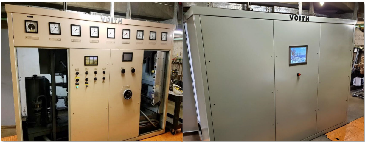
The Oxbow Power House turbine governor cabinet, before and after upgrade.
