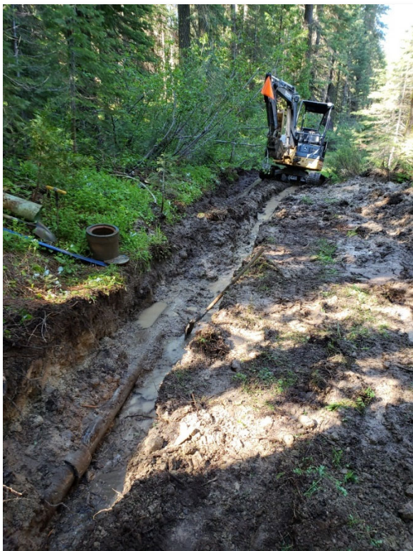
Treated Water Maintenance crews excavate to expose, identify, and make repairs to a 6-inch main line leak in the French Meadows water system.
