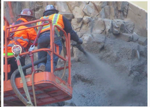
Spraying gunite on rock to prevent further corrosion
