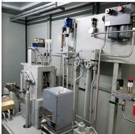
Interior of turbine governor, after modifications and upgrades.
