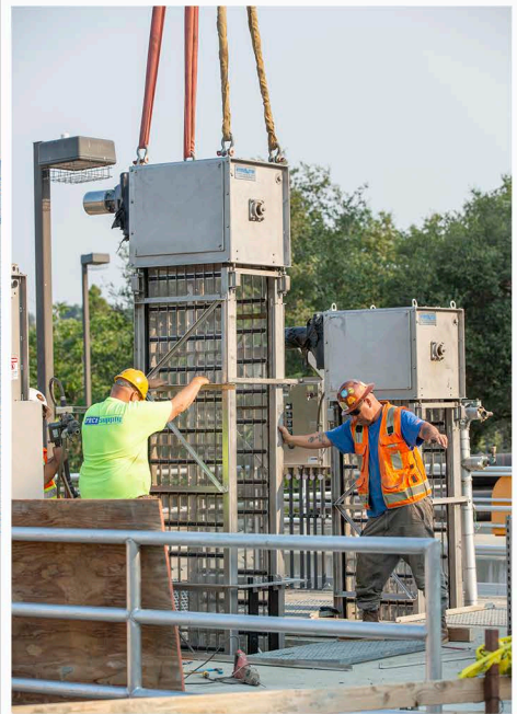
Installation of additional inlet screen.
