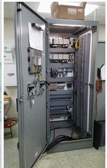
New digital controls for upgraded turbine governor.
