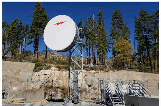
LL Anderson Dam communications tower and microwave dishes
