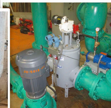
New auto backflush strainer
