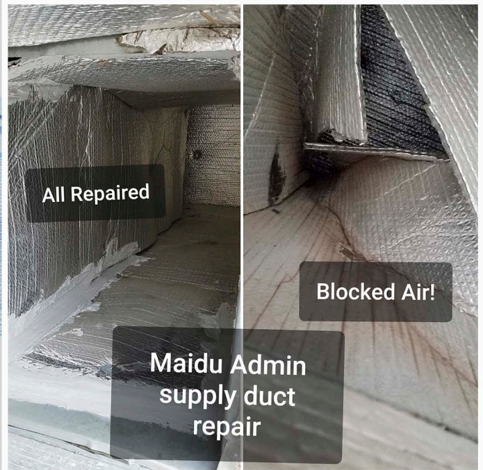
Facilities Maintenance staff unblocks supply duct at Maidu.
