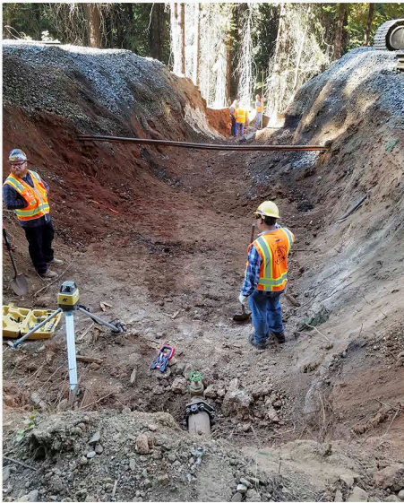
Open excavation under railroad tracks, in Alta. PCWA crews working in conjunction with Union Pacific Railroad.
