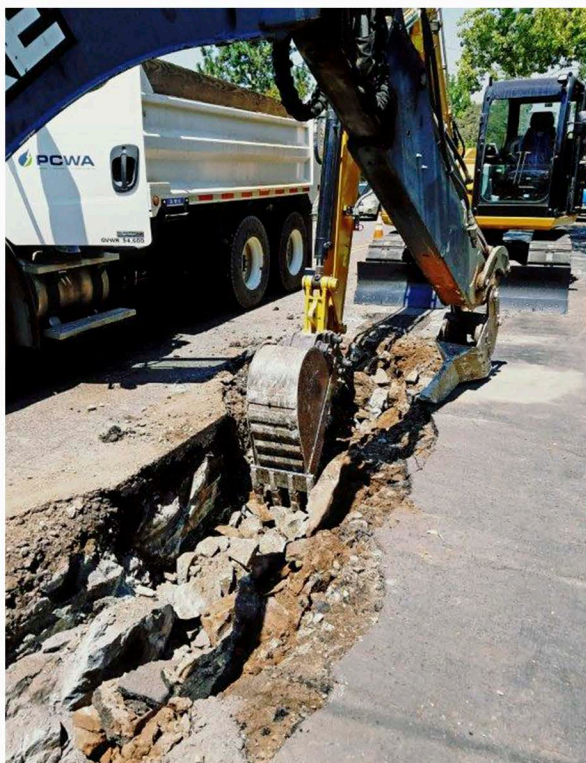
Crews using our newly purchased 308 Caterpillar Excavator and a Backhoe mounted ripper tooth to break up and excavate rock, College Way, Auburn.
