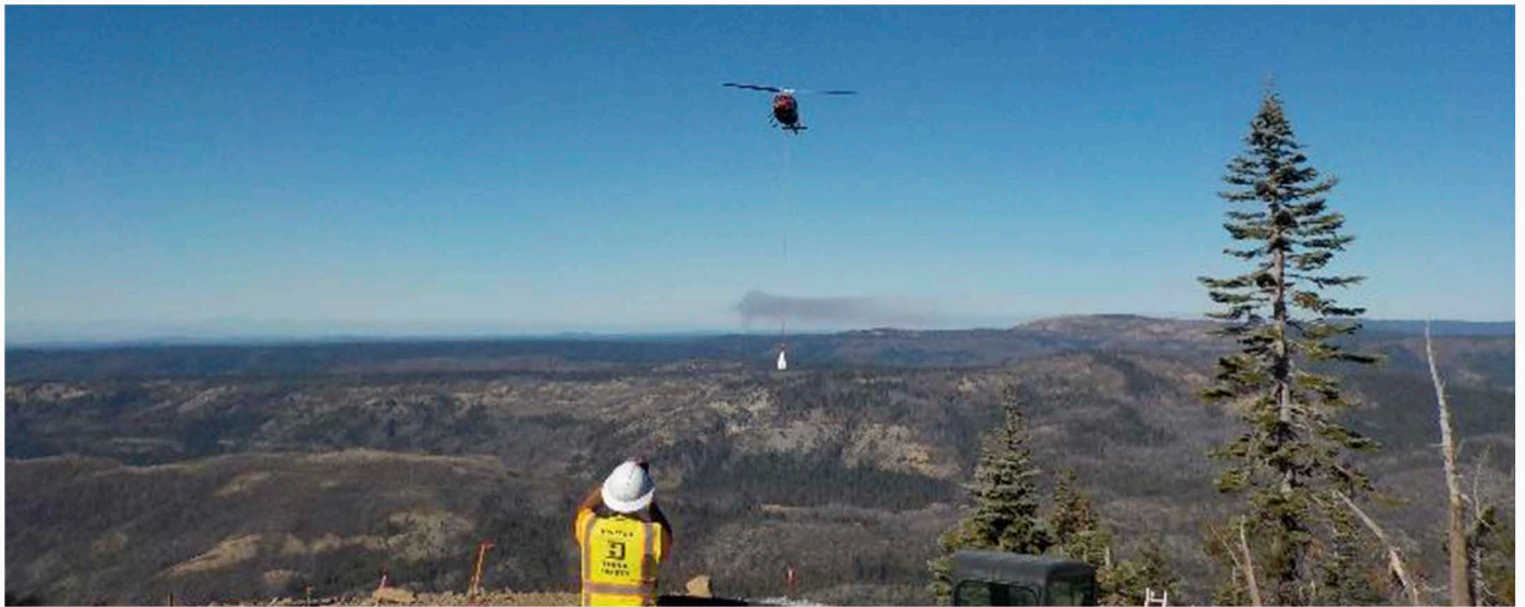
Concrete mixer trucks could not use the dirt road to the Bunker Hill Passive Reflector Site. A helicopter was necessary to fly the concrete to the site for the reflector foundation.
