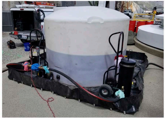
The insulating oil was reprocessed to remove contaminants and moisture.
