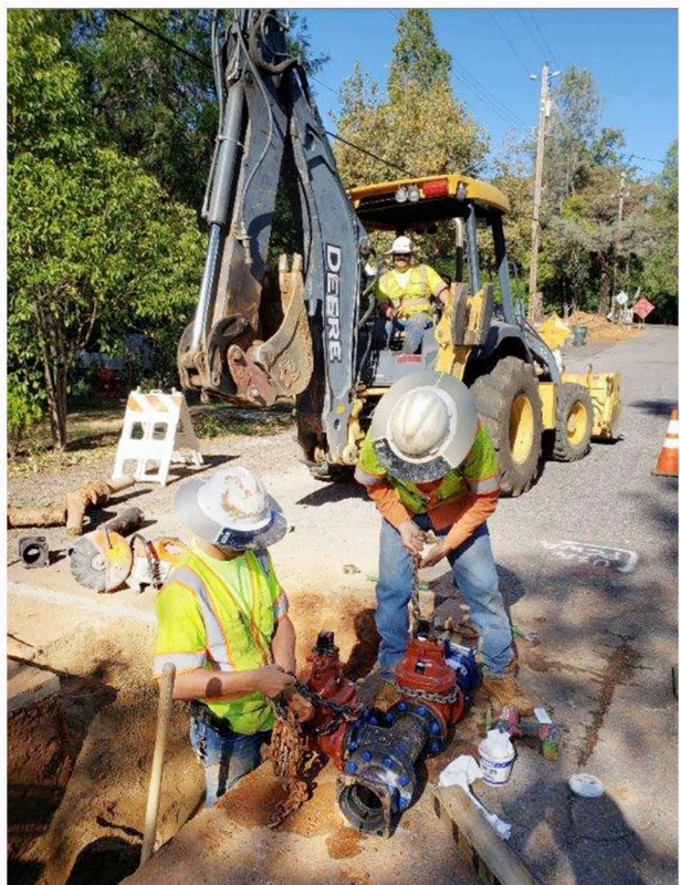
Crews assemble and prep 6-inch valve cluster prior to installation, Davis Lane, Auburn
