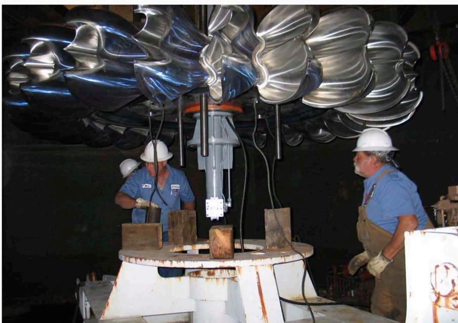
Middle Fork Powerhouse runners were replaced on Units No. 1 and No. 2 in 2010.
