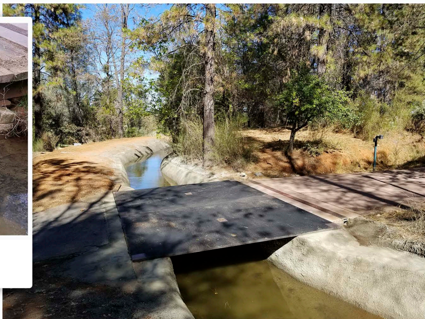
Replacement bridge over Boardman Canal in Colfax now allows full canal capacity.
