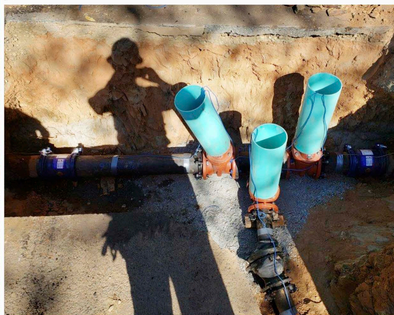
Newly installed valve cluster and tie-in points, Davis Lane, Auburn
