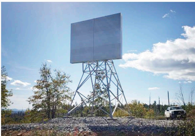
Red Star Ridge Passive Reflector Site: Construction complete.
