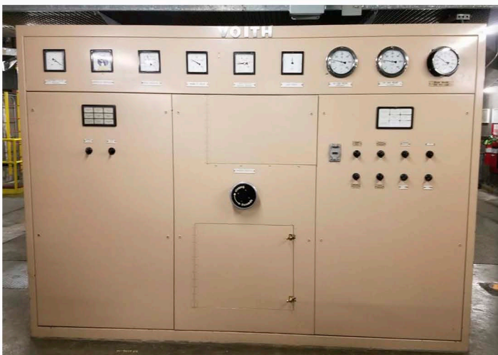
Exterior of original turbine governor cabinet, before upgrades.
