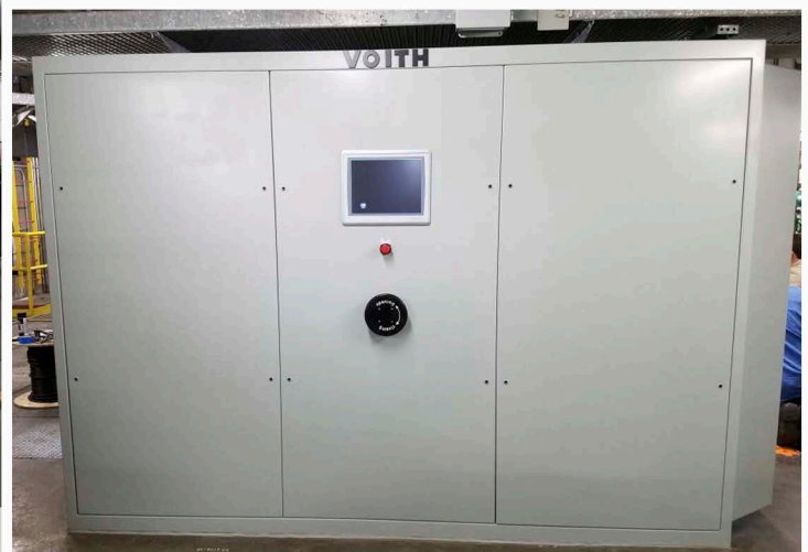
Exterior of turbine governor cabinet after modifications and upgrades.
