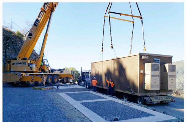
Ralston Surge Shaft communications site - setting prefabricated communication shelter
