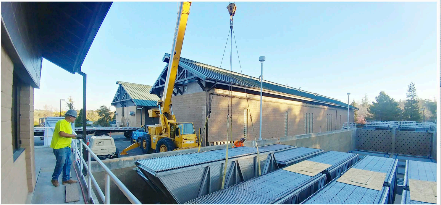
New plate settlers being installed at Foothill Water Treatment Plant No. 2.
