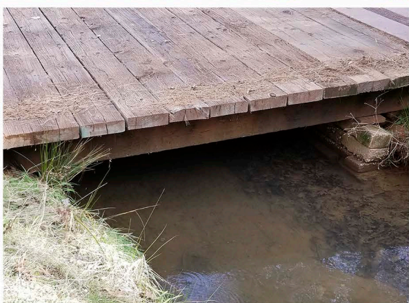
Original bridge over Boardman Canal in Colfax was failing and restricting water at higher flows.
