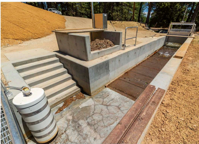
The new intake structure is equipped with fine wedge wire screens to minimize debris going through the pipe.
