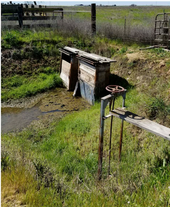
Two typical Pleasant Grove canal services before replacement.
