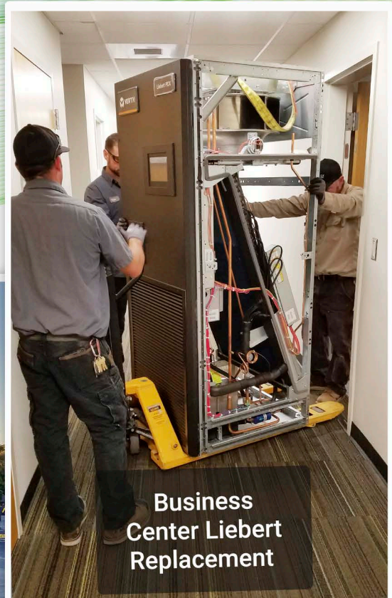
Crews move the new Liebert air conditioning unit into the server room at the Business Center.
