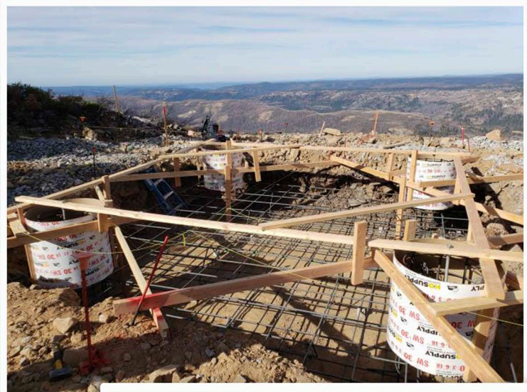
Concrete mixer trucks could not use the dirt road to the Bunker Hill Passive Reflector Site. A helicopter was necessary to fly the concrete to the site for the reflector foundation.
