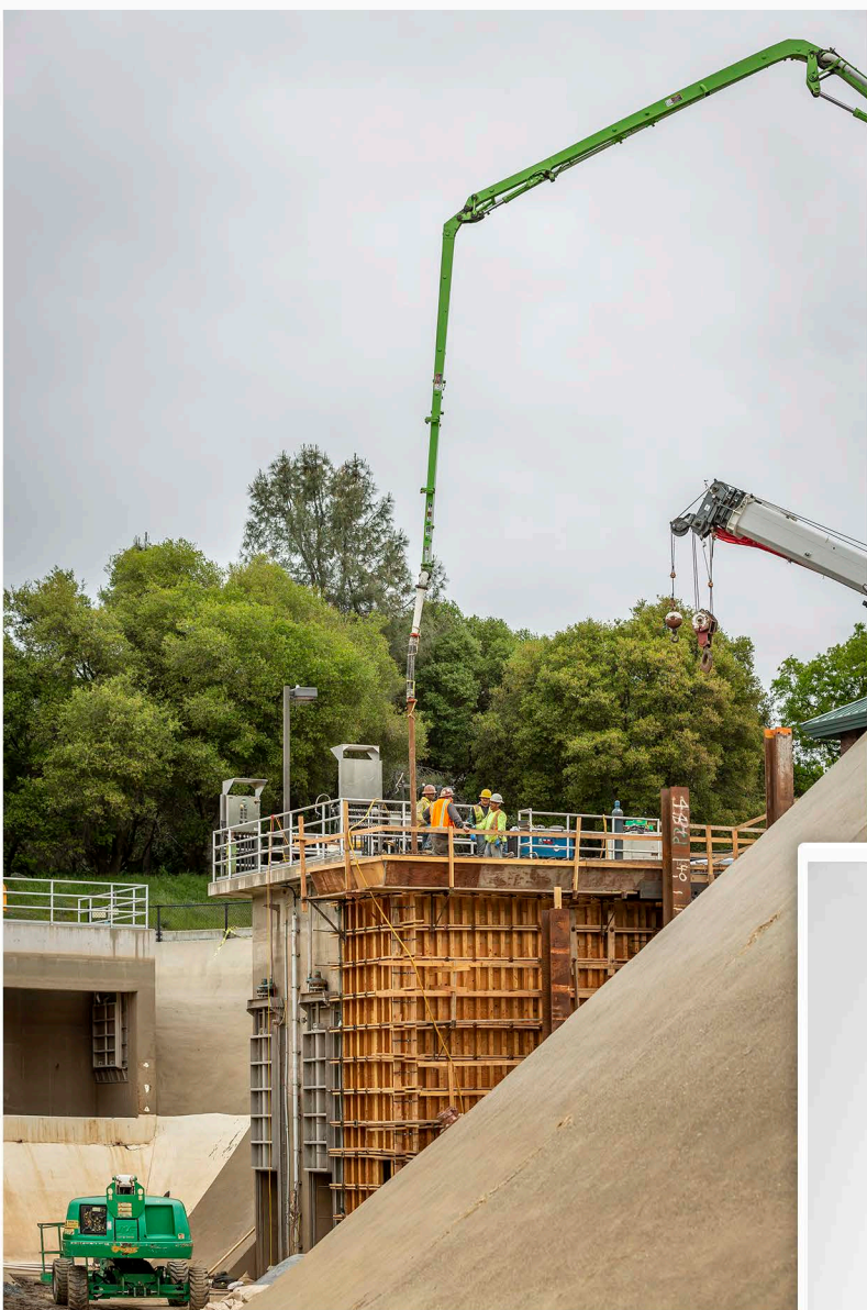
Installation of additional intake structure.
