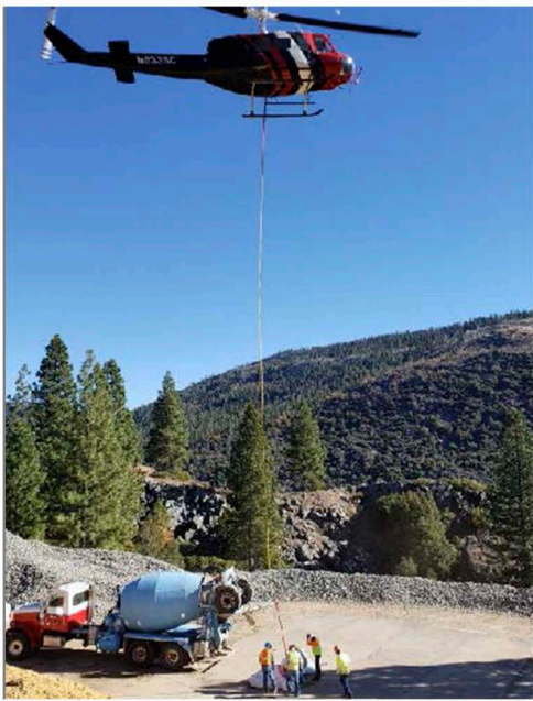
Concrete mixer trucks could not use the dirt road to the Bunker Hill Passive Reflector Site. A helicopter was necessary to fly the concrete to the site for the reflector foundation.
