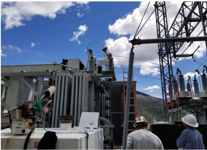
The main transformer high voltage bushings were leaking at the flange and had to be replaced.
