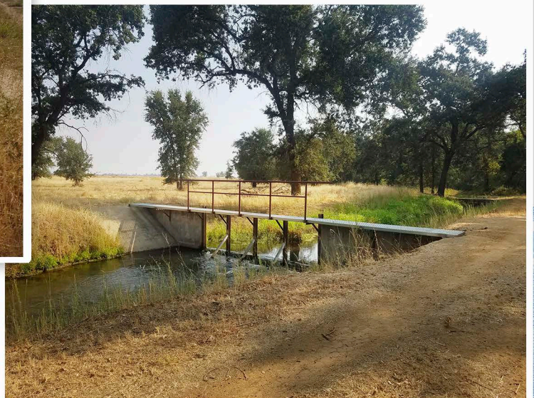
Newly fabricated metal walkways and handrailings for Canal Operator safety, Moore Canal.
