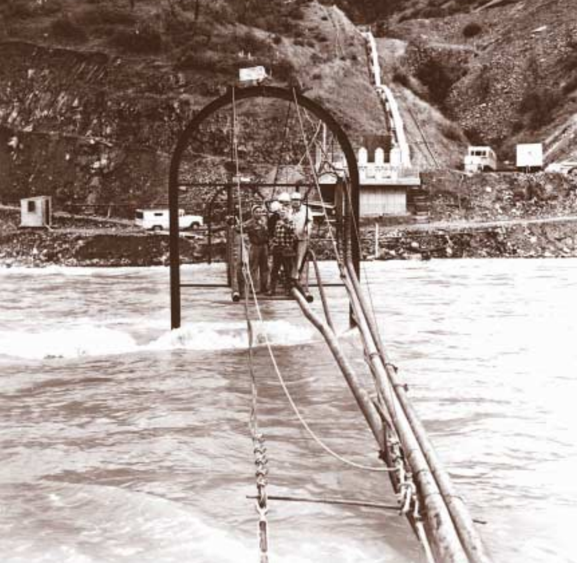
WORKERS ON THE AMERICAN RIVER PUMP STATION, WHICH THE FEDERAL GOVERNMENT REQUIRED THE AGENCY TO ABANDON WITH CONSTRUCTION OF THE AUBURN DAM.
