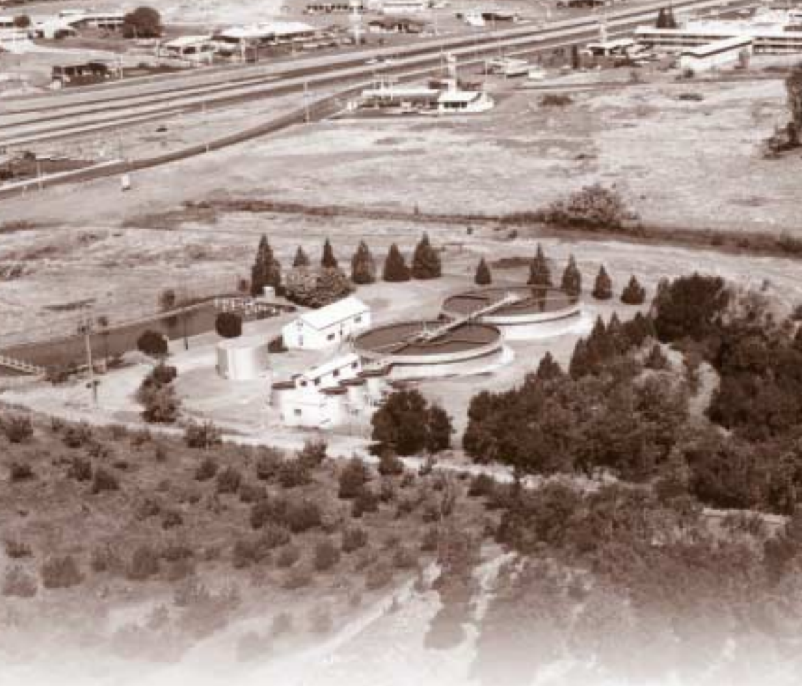
THE AUBURN WATER TREATMENT PLANT ALONG LINCOLN WAY IN THE 1960s. THE VACANT FIELD NEXT TO THE PLANT IS NOW THE SITE OF RALEY'S SUPERMARKET.
