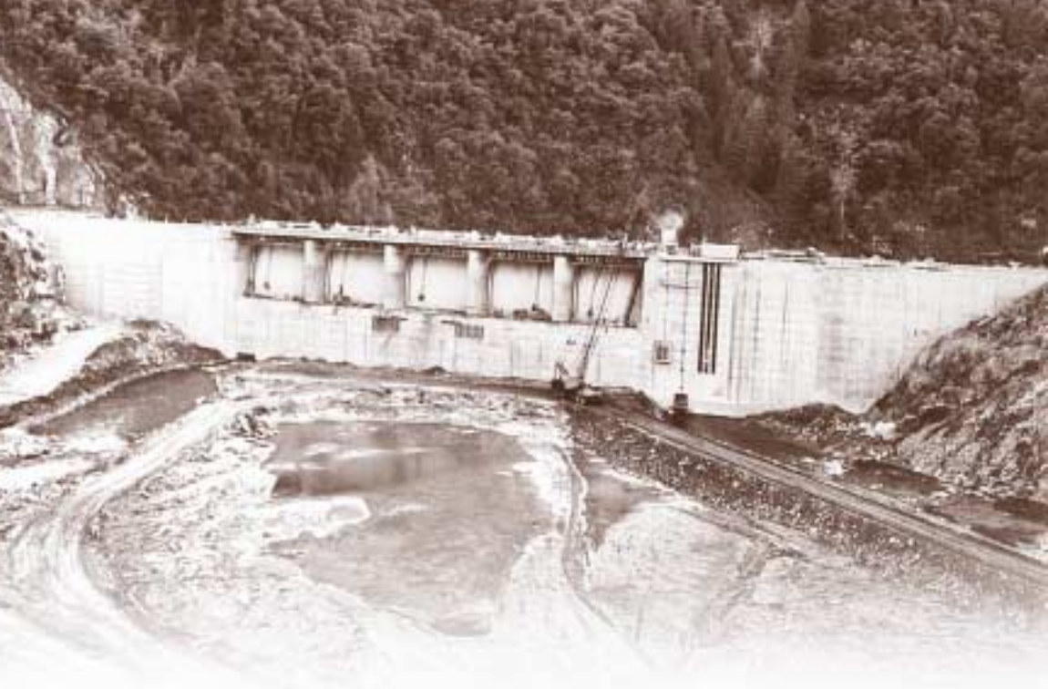
THE RALSTON AFTERBAY DAM. THE MIDDLE FORK OF THE AMERICAN RIVER AND THE RUBICON RIVER FEED INTO THE SITE.
