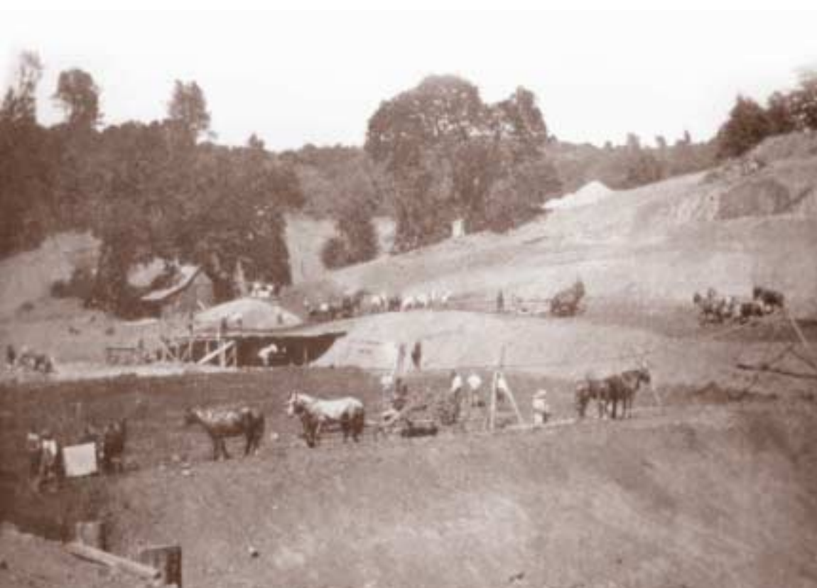
LAKE ARTHUR DAM DURING CONSTRUCTION.
