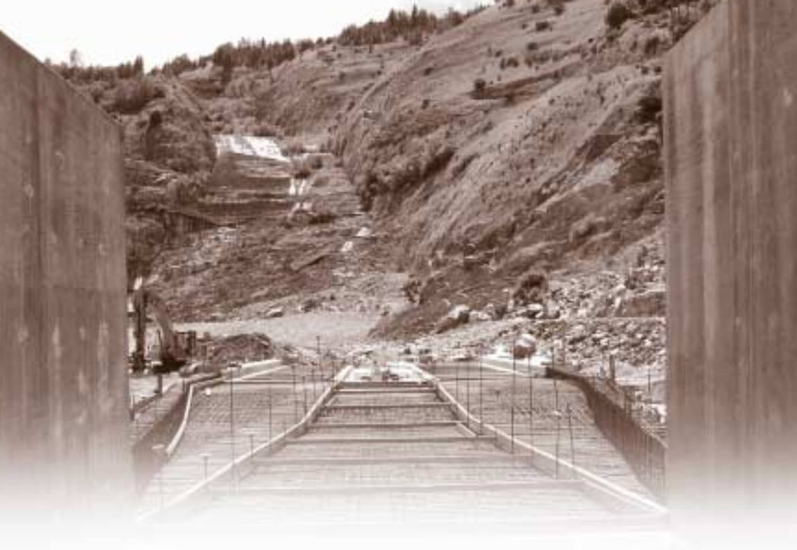
WORK ON THE NEW AMERICAN RIVER PUMP STATION BEGAN IN 2003.
